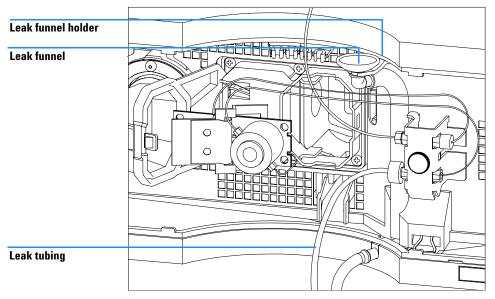
Figure 32 Replacing Leak Handling System Parts
