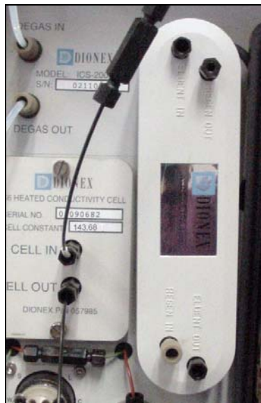
Figure B-23. Suppressor Installed (SRS Shown)
